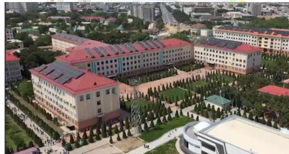
Figure 2: Location of on-grid solar systems.
