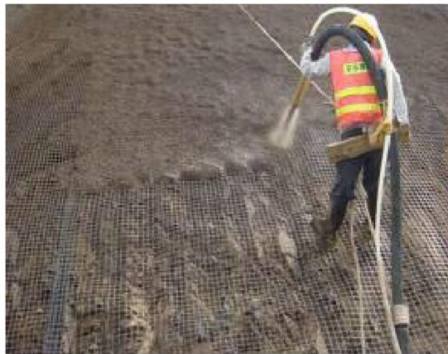
Figure 2.54 Construction methods of the living wall
