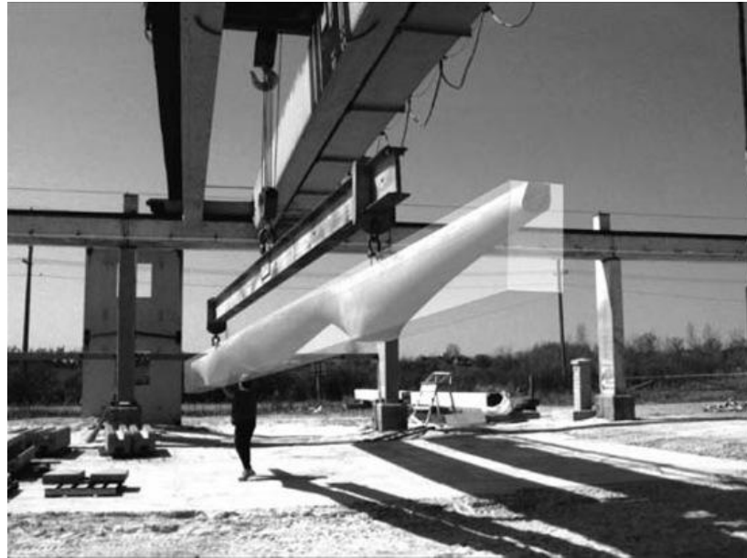
Figure 4.1 – Fabric Formed Beams, by Mark West
