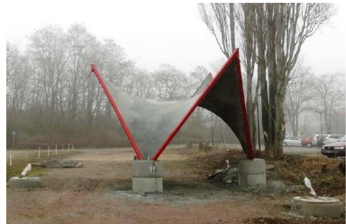
b) Constructed Membrane-Concrete Shell Prototype – March 2014
