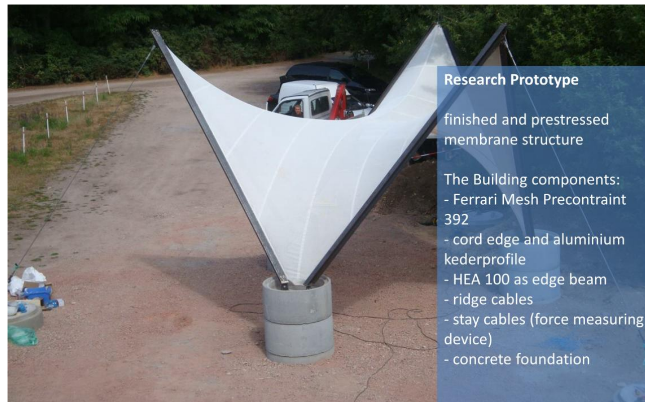
Prototype of a Fabric-Formed Thin Concrete Shell Canopy structure built at the Bernburg Campus of Anhalt University, Germany, 2013
