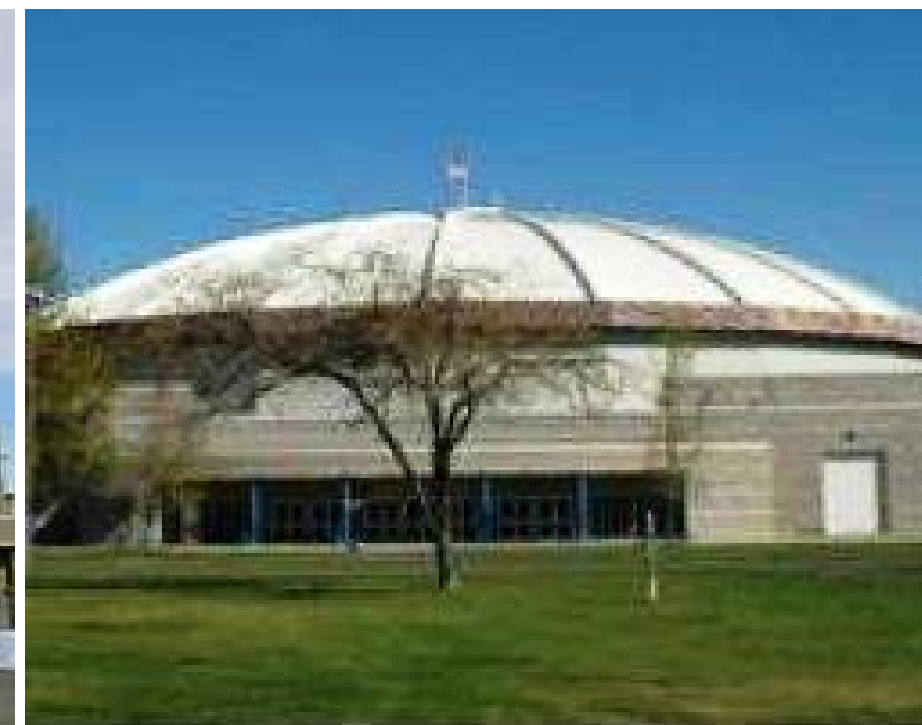
Figure 3.23 - Loofburrow Architects; J. Christiansen Engineers – 1990; Yakima, WA – USA; R = 248 ft., t = 3.75'' – R/t = 794 .
