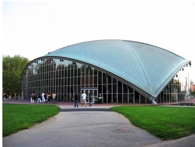
Figure 3.21 - Eero Saarinen & Associates, Architects – Ammann & Whitney – 1955; Cambridge, MA – USA; R = 112 ft., t = 3.5'' – R/t = 384 .
