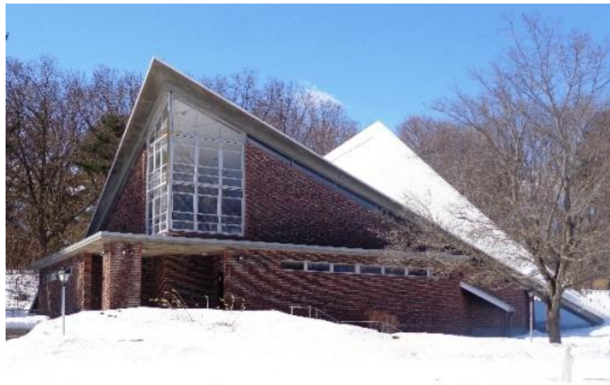
Figure 3.29 – St. Athanasius Church Hyperbolic Paraboloid Roof – Exterior Elevation Views of hypar concrete roof.
