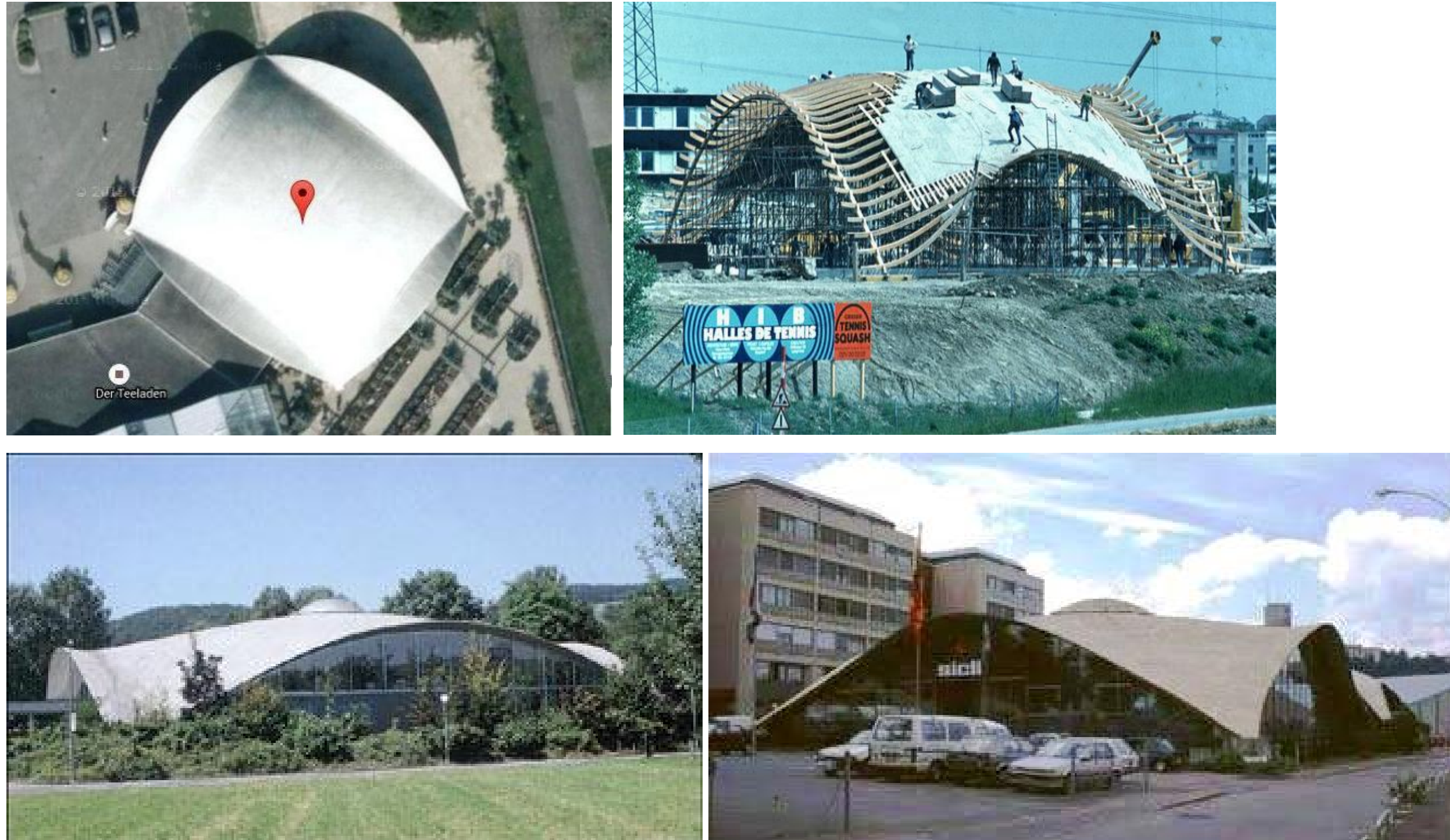
Figure 3.45 – Heinz Isler thin reinforced concrete shell projects built in Switzerland and Europe, Aerial Views, Elevations and Formwork.
