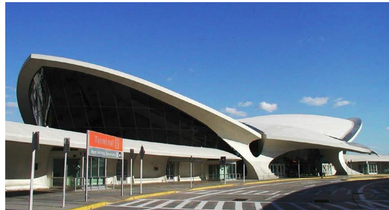
Figure 3.36 – Cantilevered Shells for the TWA Terminal at JFK Airport, by E. Saarinen, Architect, Ammann & Whitney, Engineer, NY 1962.
