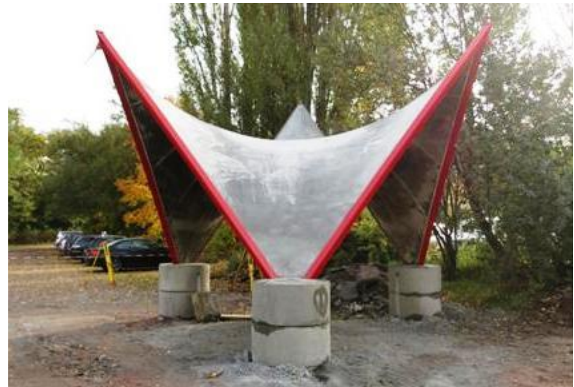
Prototype of a Fabric-Formed Thin Concrete Shell Canopy structure built at the Bernburg Campus of Anhalt University, Germany, 2013
