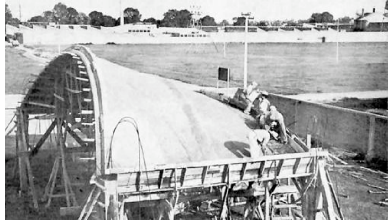
Figure 1.13 – Typical Conoidal Ruled Surface - Experimental Conoidal Roof in San Bartolo, Mexico, by Felix Candela, 1950.
