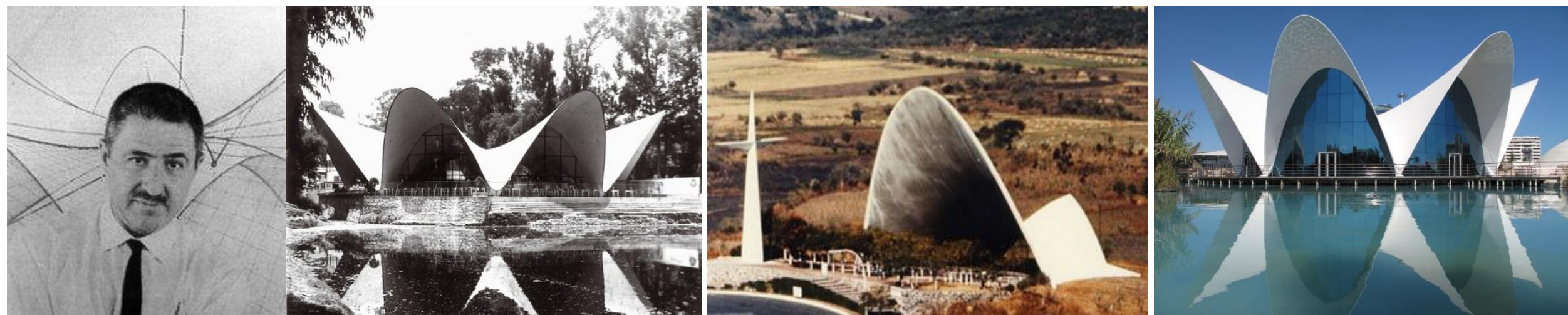
Figure 2.9 – Felix Candela and some of his hyperbolic paraboloid shell structures in Mexico and Spain.
