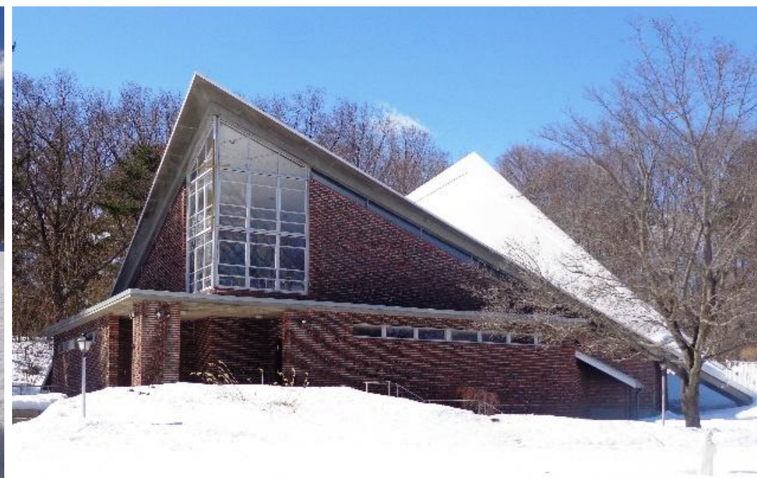
Figure 3.30 – St. Athanasius Church Hyperbolic Paraboloid Roof – Exterior Front and Side Elevation Views of hypar concrete roof.
