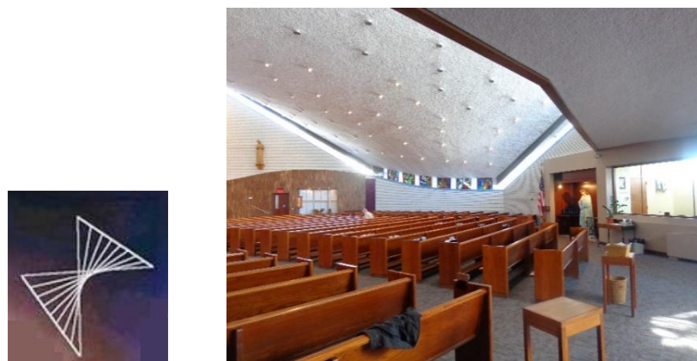
Figure 3.28 – St. Athanasius Church Hyperbolic Paraboloid Roof Aerial View, Rendering, and Interior view of hyper concrete roof.
