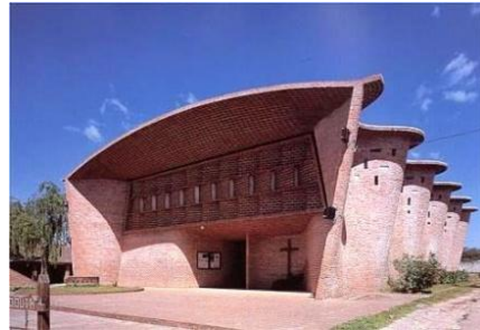
Figure 1.14 – Church of Christ the Worker, Floor Plan and Exterior Conoidal Reinforced Brickwork, by Eladio Dieste, Atlantida, 1960.
