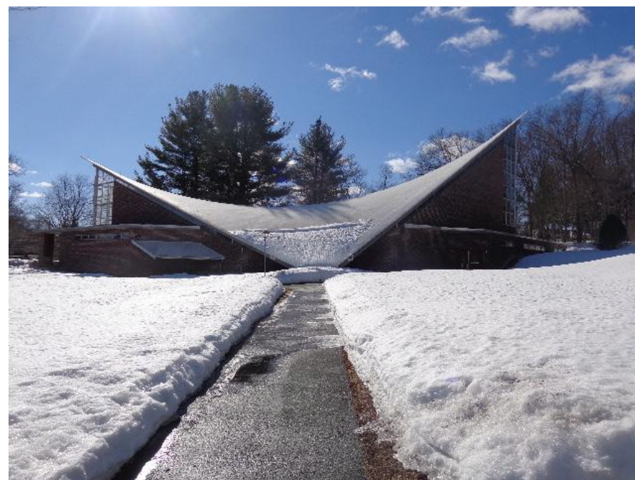
Figure 3.30 – St. Athanasius Church Hyperbolic Paraboloid Roof – Exterior Front and Side Elevation Views of hypar concrete roof.
