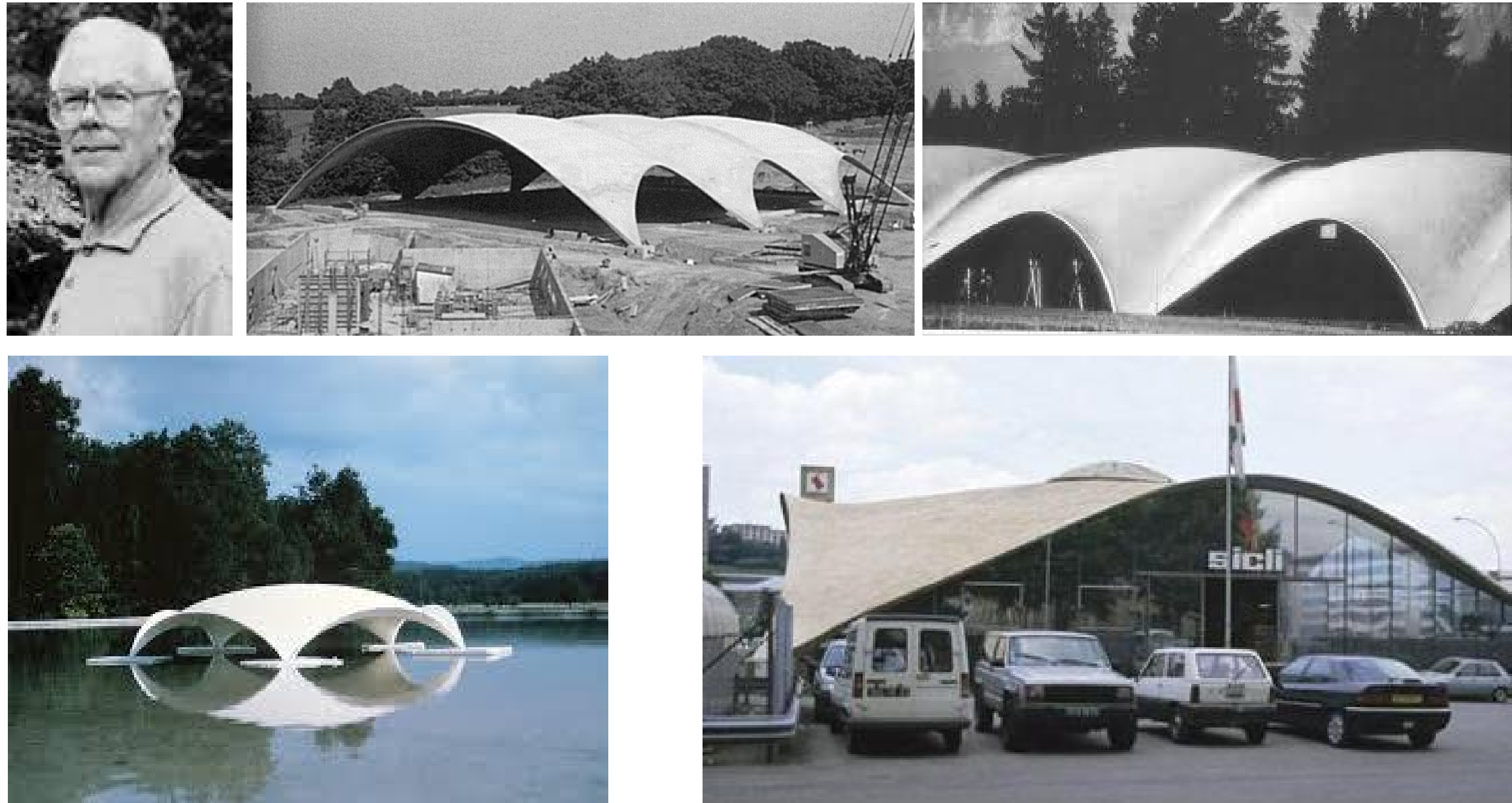
Figure 3.42 – Heinz Isler and some of his constructed thin reinforced concrete shells in Switzerland, Europe.
