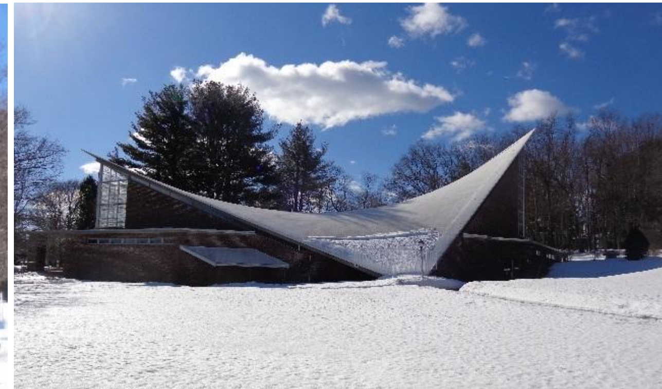
Figure 3.29 – St. Athanasius Church Hyperbolic Paraboloid Roof – Exterior Elevation Views of hypar concrete roof.
