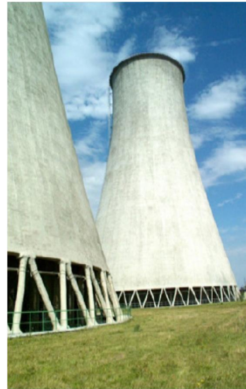
Cooling Towers, Europe
