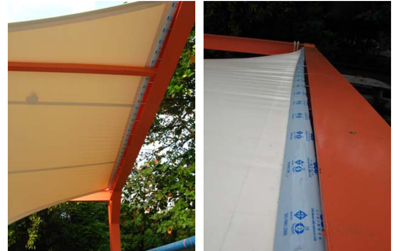
Figure 4.5 Clamping Plate Edge (I)
