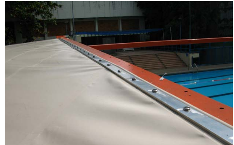
Figure 4.6 Clamping Plate Edge (II)
