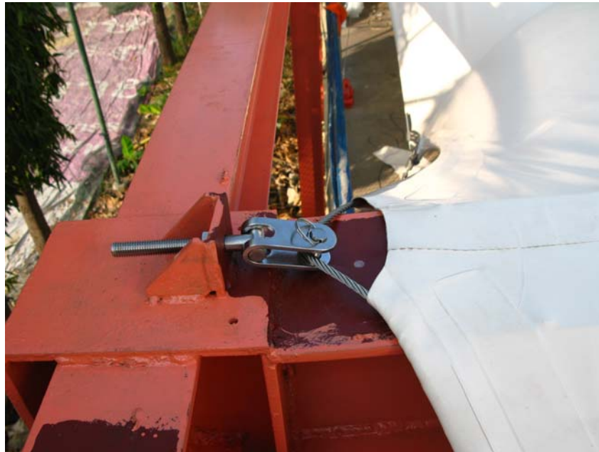
Figure 3.2 Boundary cables and Thread toggle
