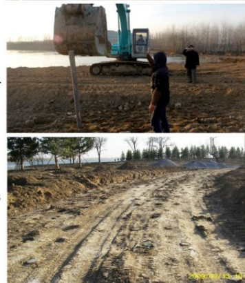
Fig. (48) The lakefront: was stabilized, load-bearing capacity was increased, and roads were constructed using waste plant materials and coal ash, Source: LPS-CSB- 494, 2012; Beijing Tsinghua Urban Planning & Design Institute; Biennial, An, Y., et al., 2014
